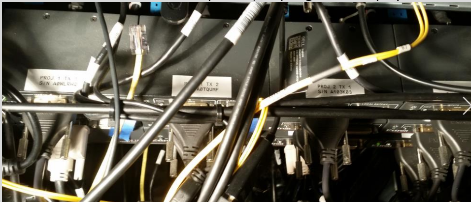
Render node USB extension endpoints (Output goes to DisplayPort's of render node GPUs).
